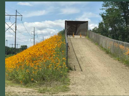
Ashuelot Rail Trail, South Bridge, Keene
