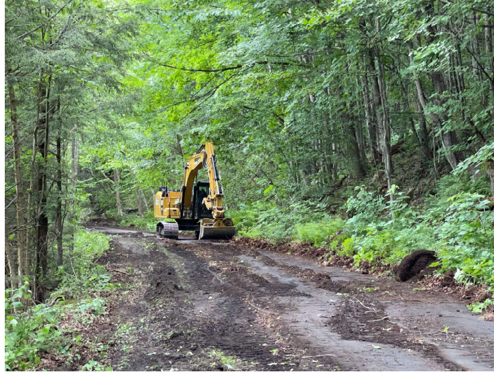
During: Ditch, Grade, Crown
