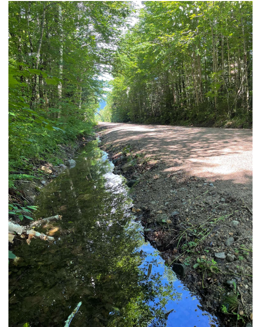
After: Water flows down the ditch
