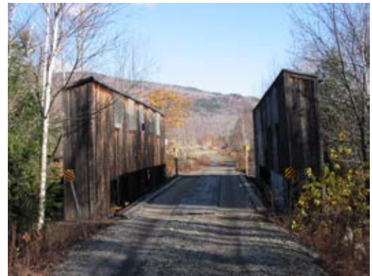
Boxed Pony Truss Bridge on Rail Trail
