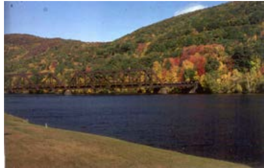
Rail bridge over Connecticut River
