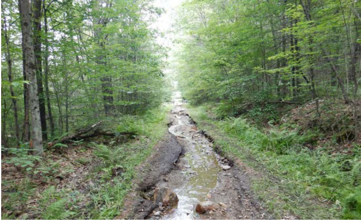
Storm damage on the Cheshire Rail Trail.
