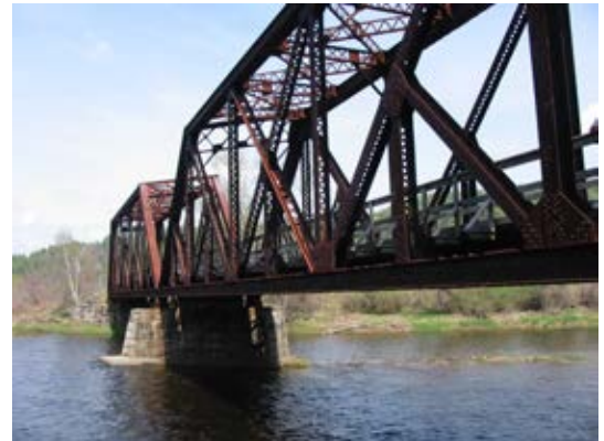
Rail bridge over Ammonoosuc River in Lisbon
