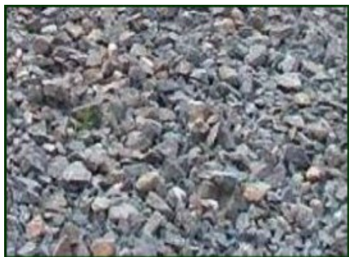
Ballast rock surface
